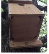
View showing recessed floor with corner cutouts for drainage
